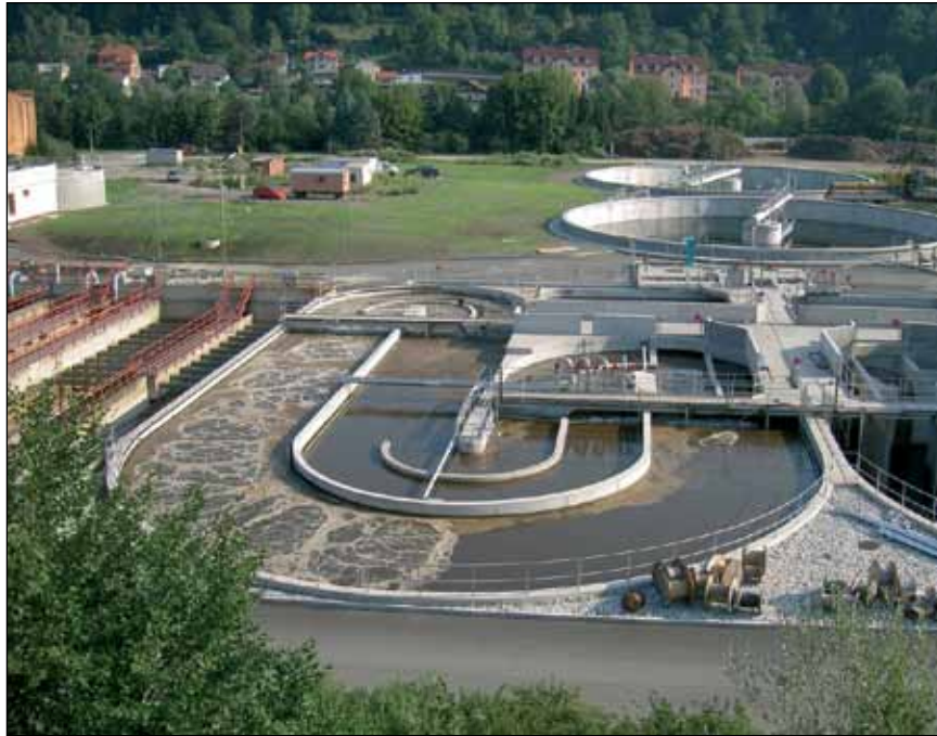
Hauptkläranlage is Vienna's major waste water treatment plant in the low-lying district of Simmering. Much of Vienna's sewage system uses gentle gradients, so little pumping is required to get the waste to its destination.
