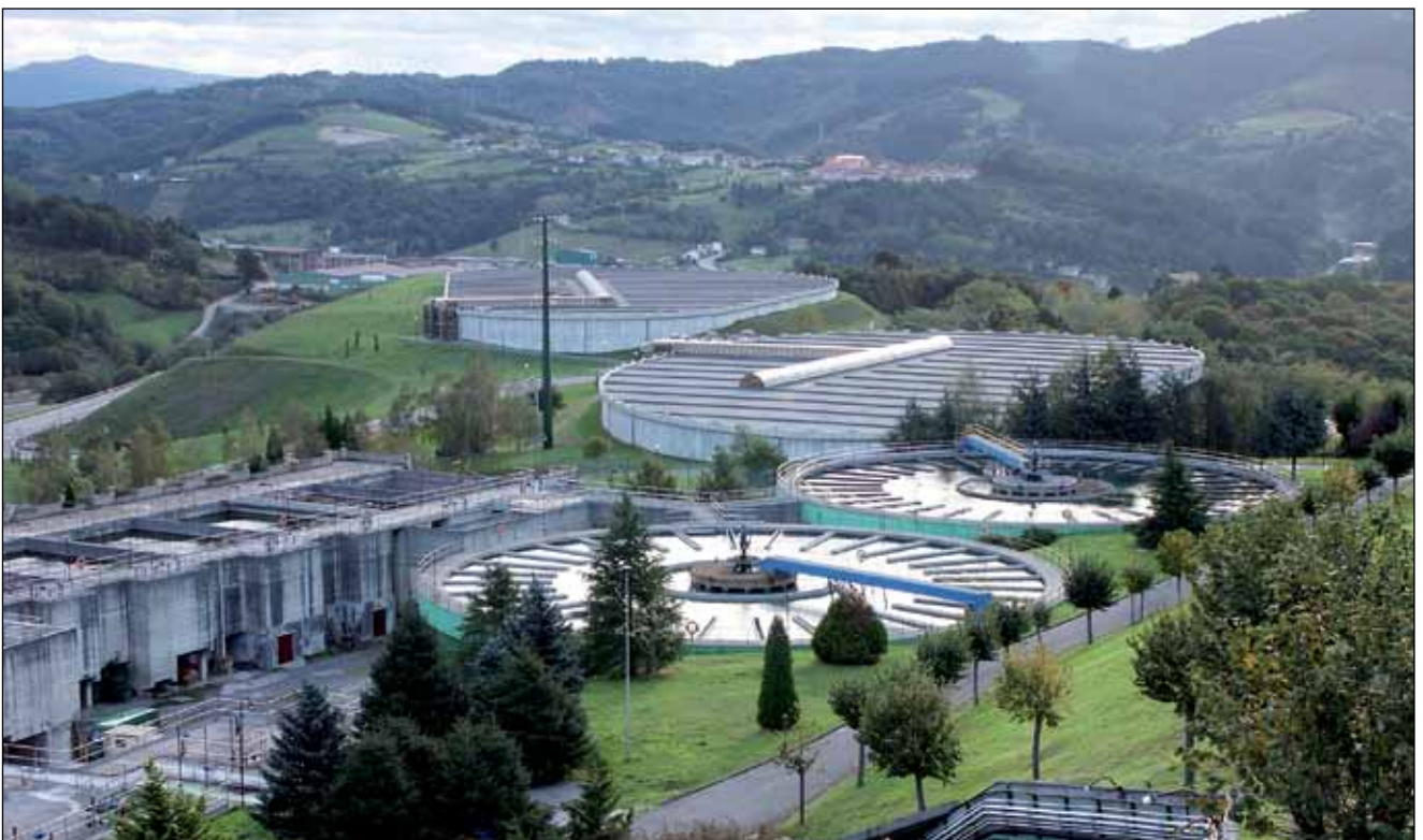
The water purification plant at Venta Alta in Arrigorriaga, Bizkaia is one of Spain's largest water treatment plants, with a capacity of 7m 3 a second.
