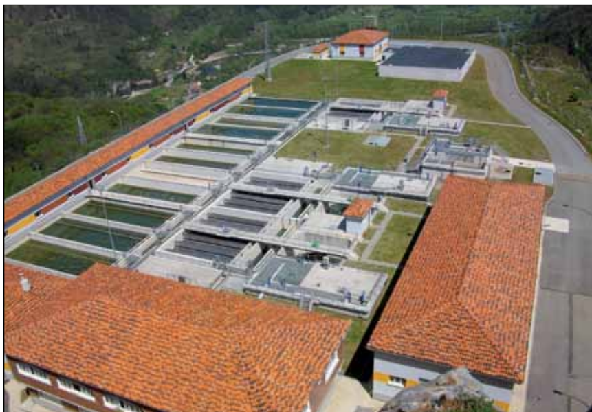
The Áramo Quiros waste water treatment plant at Oviedo in Spain has been built in a mountainous region and serves 300.000 people. Construction was completed in 2010.
