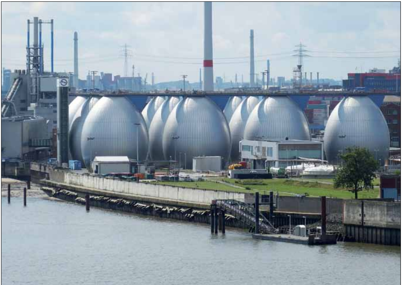
The Hamburg Water Cycle project in Germany treats separate streams of waste water: blackwater (from toilets), greywater (kitchen use, showers, etc) and rainwater.
