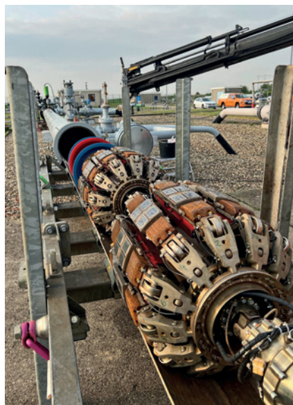
During the status analysis of existing pipelines within the scope of the project, a special measuring probe to determine crack-like defects was tested for the first time.
