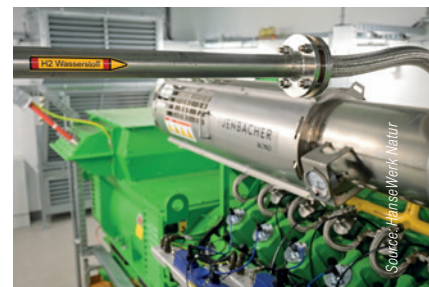
The gas motor by INNIO in Jenbach was temporarily converted for the field test.
