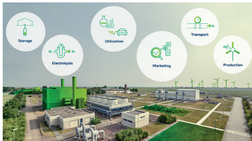
The Energy Park Bad Lauchstädt is a regulatory sandbox for the generation and use of green hydrogen.
