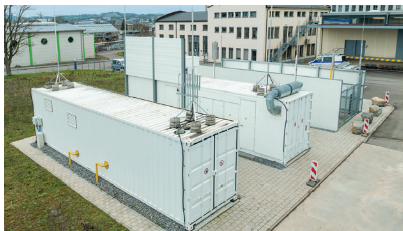
System layout (from the right): spare storage, electrolyser and blending system (inside the container)
